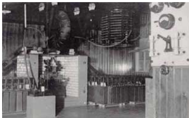
Figure 3: Clifden, Ireland condenser under construction. (Marconi Company)
