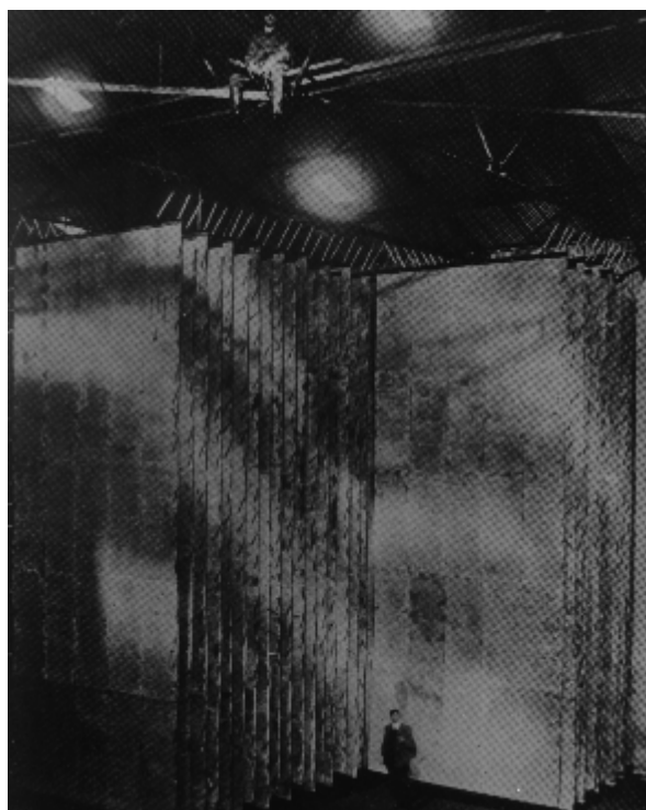
Figure 3: Clifden, Ireland condenser under construction. (Marconi Company)
