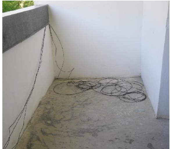
Counterpoises of the Balcony Vertical HF Antenna
