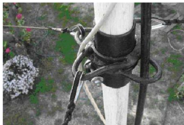
Picture 3 Jointing Mast's Tubes
