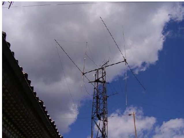
Figure 2 Antenna Mast with the All- Metal Three Element Antenna
