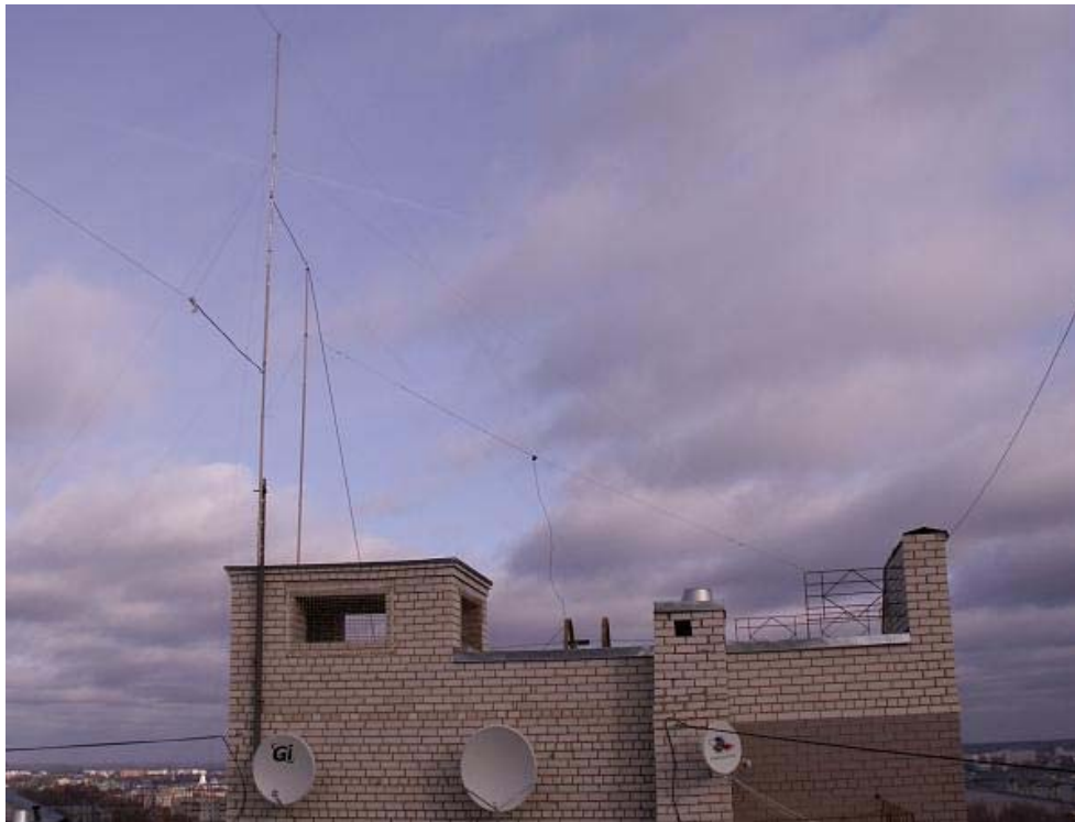
Figure 5 Antenna Strela on the roof
