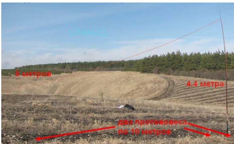
Figure 3 shows the antenna installed in Caucasus Mountains
