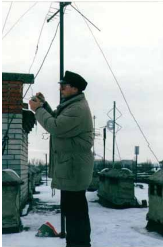
Photo: Finding of resonance of the guys with help a GDO
